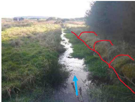
Fig. 5: View downstream of Channel 2. Straightened and slow flowing. Stone embankment on the right hand bank (in red) preventing lateral movement of the channel. Recommendation - removal of right hand bank embankment and installation of wood and brash structures would give more sinuosity and encourage water retention.
