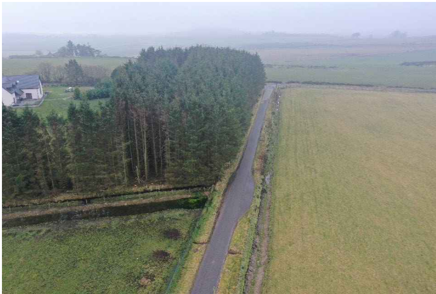
Figure 2 Aerial view of ponding at drainage outfall
