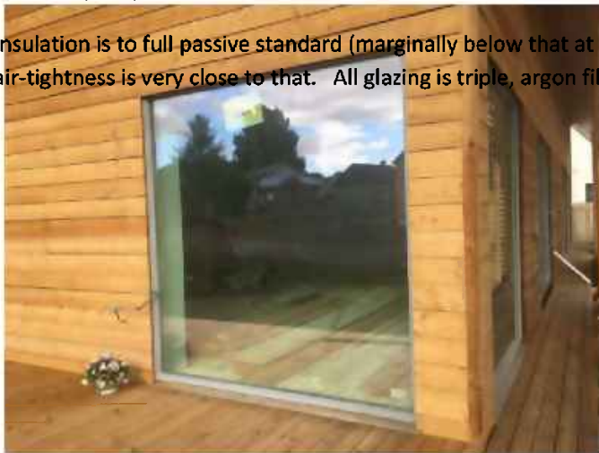
Larch cladding detail – Model D4 house at Auchleven
